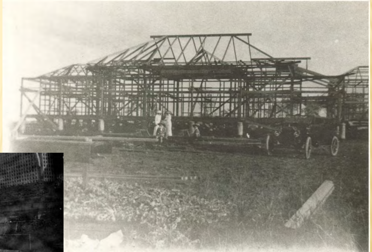
Greenmount under construction
