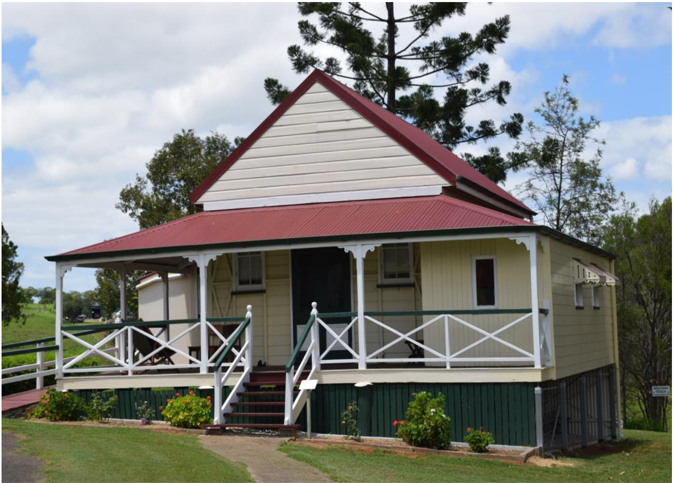
Image Caption: The Goolman building, half of the original Goolman Divisional Board building prior to the Shire name change to Boonah Shire.
